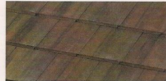
Flat Tile Roofing: Saxony 900- Chestnut Burnt
